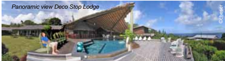
Panoramic view Deco Stop Lodge
